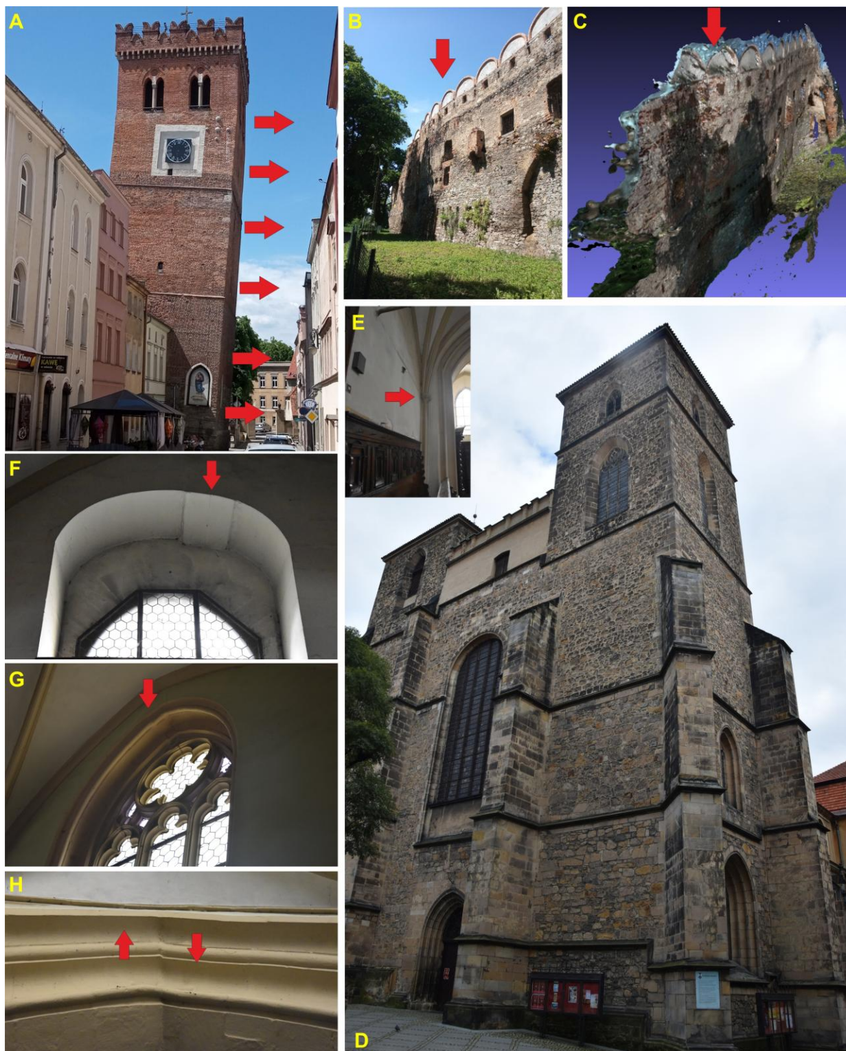
Figure 1. Examples of observed deformation/restoration suggesting seismic origin. A – Leaning Tower in Ząbkowice Śląskie presenting >2 m deviation from the vertical; B & C – Castle in Ząbkowice Śląskie with folded wall (fold with subvertical axis); D-H – Church of the Assumption of the Blessed Virgin Mary in Kłodzko; D – general view on the exaggerated buttresses supporting two uneven towers and NW wall; E – tilted inward NW wall; F – dropped keystone above the portal on the NW wall; G – dropped and shifted keystone above window in SW wall; H – deformed arch below N tower.
