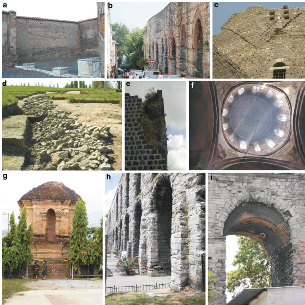
Fig. 2 (a) Arcuate out-of-plane collapse in the market, Pompeii, Italy, repaired before the 79 AD eruption of Vesuvius, which buried the city. Photo: Kázmér #9266. (b) Warped northern side of the Valens aqueduct (Istanbul, Turkey). Completed in 368 AD, several subsequent earthquakes left their traces on the massive construction #0340. (c) V-shaped damage on the SW wall of the twelfth-century donjon of al-Marqab citadel, coastal Syria. The damage was inflicted by the 1202 earthquake (Kázmér and Major 2010) #4589. (d) Fallen masonry fence in the Roman city of Carnuntum (Deutsch-Altenburg, Austria) #5496. (e) Triangular missing parts in corners of walls (al-Marqab citadel, coastal Syria) #4671. (f) Deformed circular dome of fourth- to eleventh-century Samtavro cathedral, Mtskheta, Georgia #1633. (g) Tilted Buddhist stupa (approximately fifteenth century) in Chiang Mai, Thailand. While a single tilted building does not indicate seismic origin, this stupa is one of 21 sites displaying tilting in the city (Kázmér et al. 2011) #3411. (h) Buttresses support the pillars of the Valens aqueduct in Istanbul, Turkey, completed in 368 AD #0335. (i) Valens aqueduct in Istanbul, completed in 368 AD. A brick arch was built to support the weakened stone arch after one of the frequent earthquakes in the region (Istanbul, Turkey) #0335
