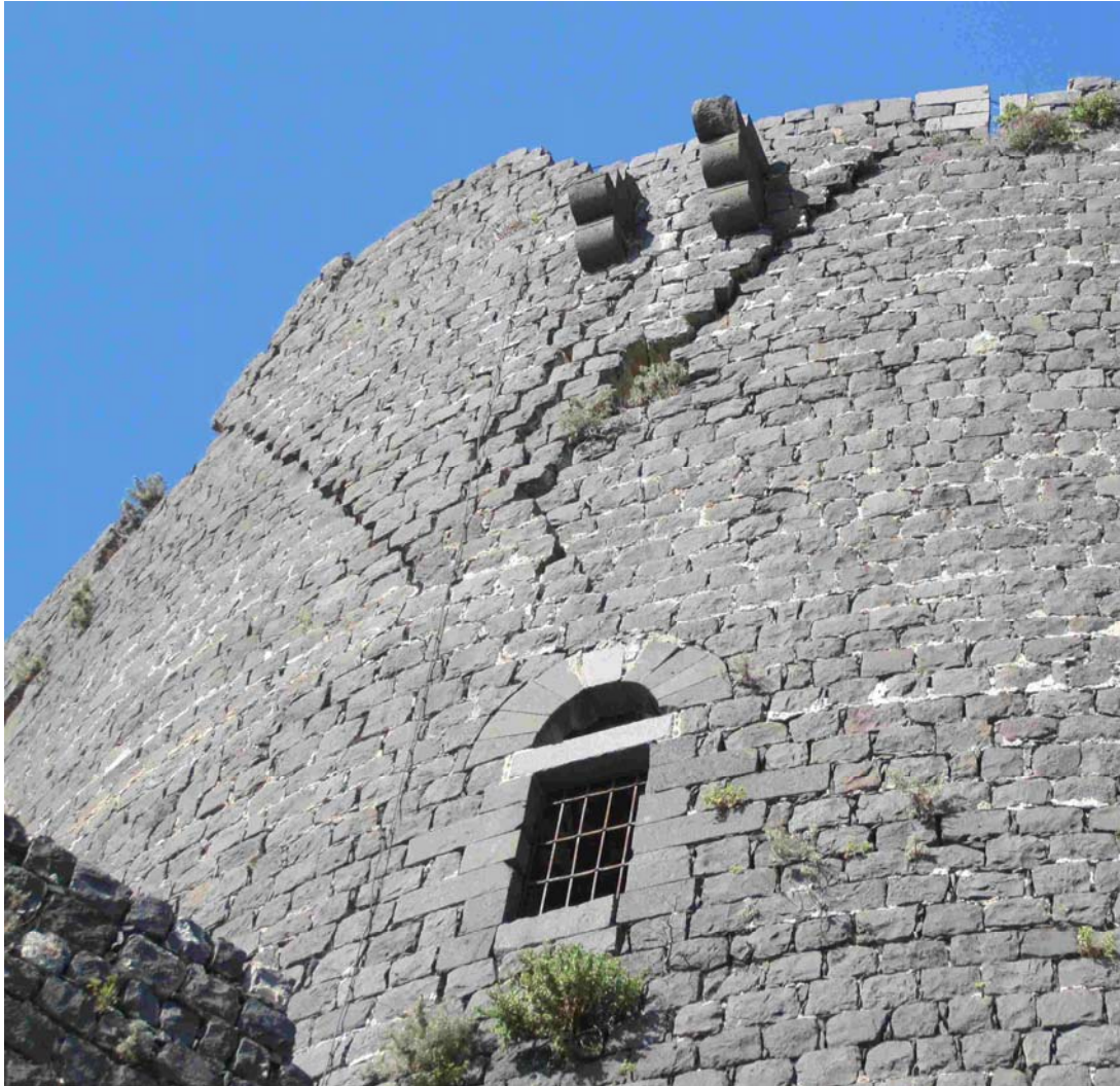
Fig. 6.52. V-shaped, extruded block bordered by conjugate faults. A wedge-shaped block of masonry, ca. 7 \times 7 m, shifted toward 240^\circ azimuth by \sim 20 cm during the largest known earthquake in the Near East, in 1202 AD. Donjon of al-Marqab citadel, Syria, built by the Hospitaller knights in late 12th century. Built of Roman concrete (rubble in lime), the external and internal walls are faced by dressed basalt blocks. Walls are up to 5 m thick, diameter of the tower is 20 m. Between floors – where the extruded wedge is – the building is compact. Al-Marqab, south of Baniyas on the Mediterranean coast, Syria ( 35^\circ 09' N , 35^\circ 56' E ). Photo #1798.
