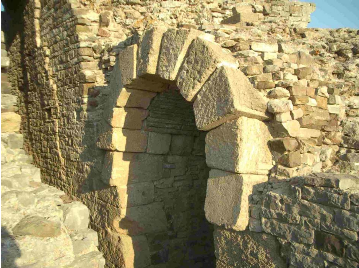
Fig. 6.53. Distributed left-lateral strike-slip deformation in the Roman theatre of Baelo Claudia, Gibraltar Straits, Spain ( 36^{\circ} 05' N , 5^{\circ} 46' E ). There are conspicuous displacements visible on the wall of the staircase and between the blocks forming the arch in the foreground. Displacement is larger upwards (max. 10 cm), indicating seismic shaking: the top part of the building oscillated with higher amplitude than the lower part, attached to the foundation.
