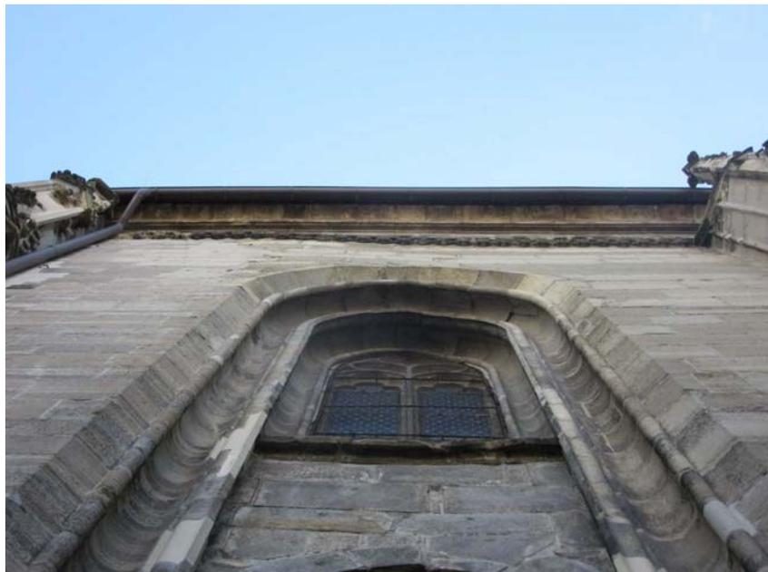
Fig. 5 - Southern wall of the apse: the upper portion above the window suffered an out-of-plane displacement. The part on the left moved towards the viewer by more than 10 centimetres. It is not a construction error: it is due to intensive shaking, perpendicular to the plane of the wall. Photo #1151
