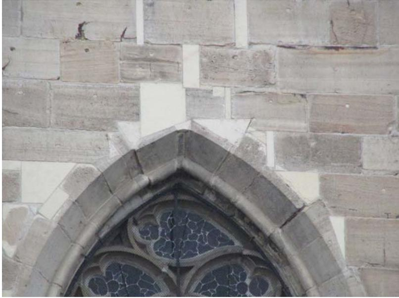
Fig 2 -.Dropped stones of the tipped arch of a Gothic window. One block on the left and three blocks on the right dropped downwards by a few centimetres during in-plane shaking of the building. White blocks are newly inserted stones to fill up empty space between shifted blocks (two upper rows) and irreparably broken blocks surrounding the window. Photo #1074
