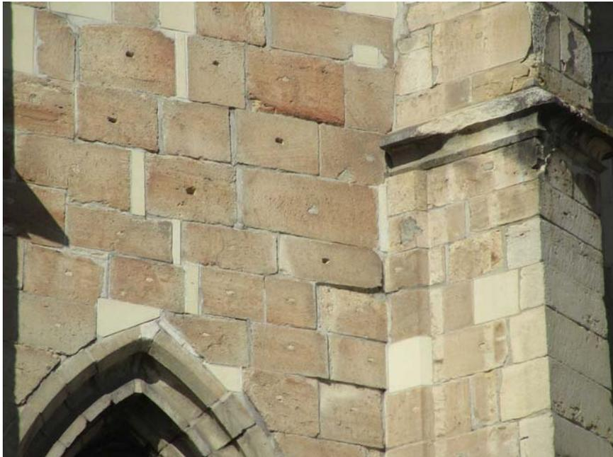
Fig 3 - Repaired traces of in-plane shift of adjacent masonry blocks (white fillings) above the Gothic window. A block adjacent to the supporting pilaster to the right has been rotated clockwise relative to the plane of the wall: its right edge is several centimetres towards the viewer. Photo #1127
