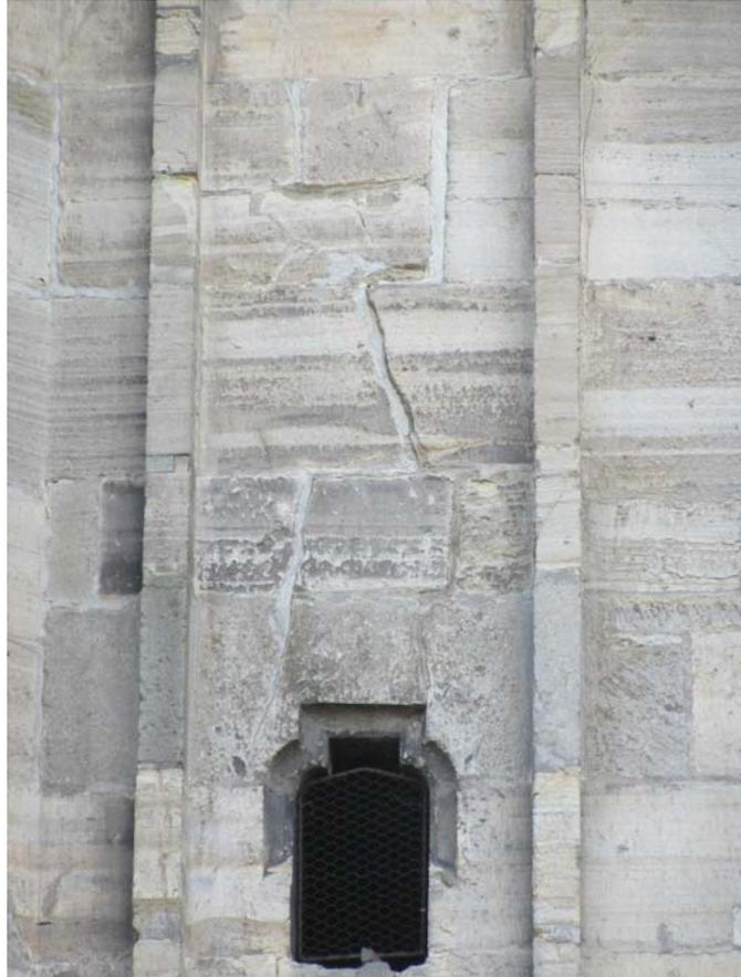
Fig. 4 - Broken ashlar in the middle of the picture window lintel broken twice. Repaired traces of stone blocks shifted in-plane. Wall of the southern aisle, window into a staircase. Photo #1139
