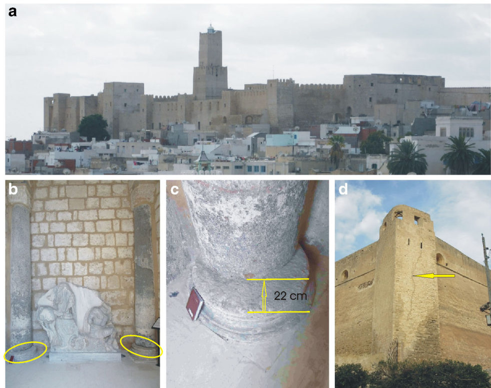
Fig. 5 Evidence for damaging earthquake affecting the kasbah in Sousse. a View of the huge fortress from northeast. #5857. b Both marble columns on the right and left are shifted on their respective plinths (encircled). #5926. I = IX. c Figure NW column at the kasbah museum entrance, shifted on the plinth by 22 cm in northwestern direction. #5928. I = IX. d Tower on the southwest corner is fractured vertically (arrow) (see also Bahrouni, 2020a: Fig. 7c). #5915. EMS98 intensity is assigned after Rodriguez-Pascua et al. (2013). 35° 49' 22" N, 10° 38' 09" E
