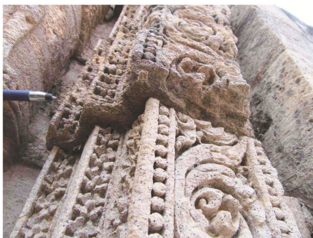
Figure 4. Shifted block in Mayadevi Temple at the Sun Temple complex, Konark, Odisha, India. Pen kept for scale. ADB Photo #2751.
